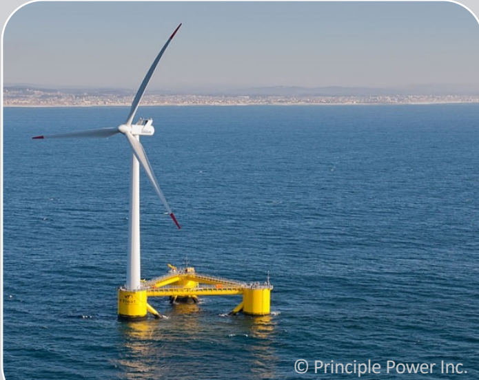
WindFloat 1 Prototype (one 2.3 MW turbine)
