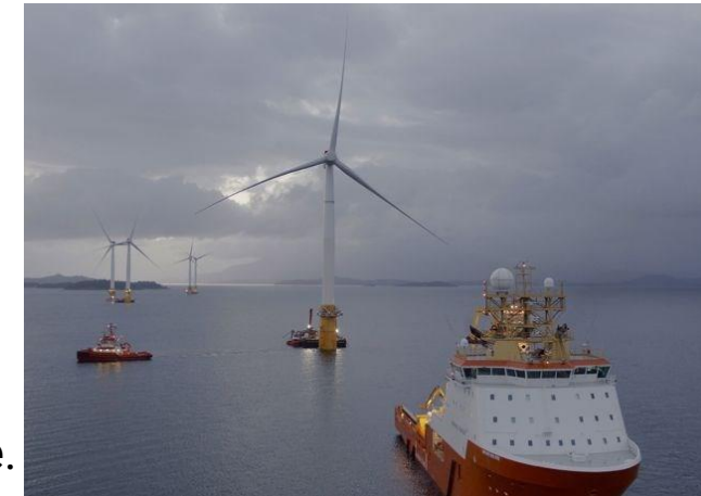
Hywind Scotland 6MW turbine being towed to site
