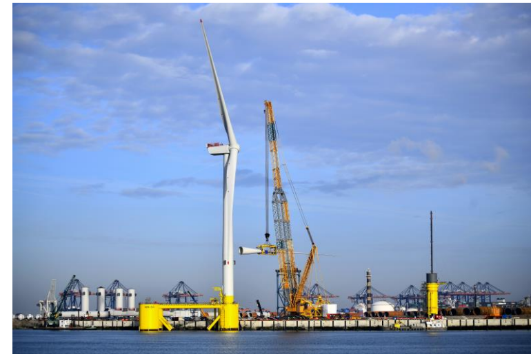
Kincardine 9.5MW turbine being installed
