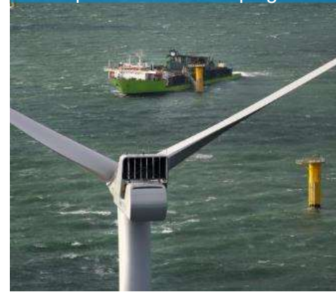
DEME – Flintstone Deepwater Rock Dumping Unit
