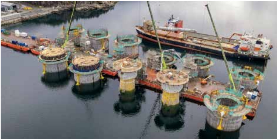
The Hywind Tampen concrete TLP substructures nearing completion. Photo courtesy of Kvaerner.
