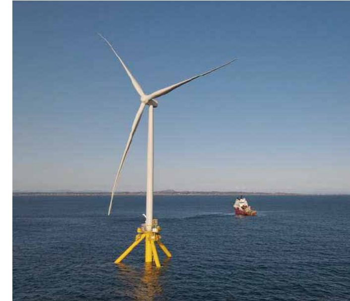
The next step in developing commercial scale: the modular-built TetraSpar in full scale demo, offshore Norway (2020).
