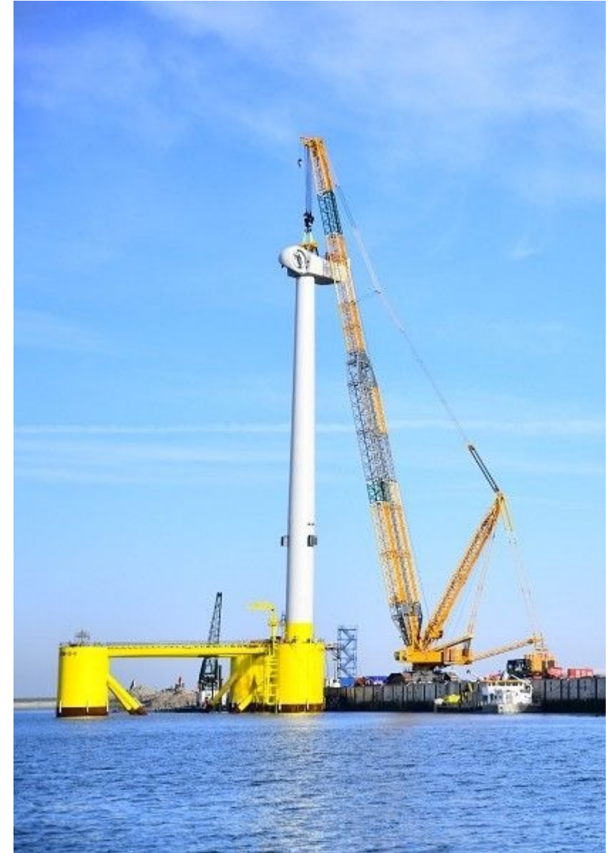
V164-9.5MW WTG being installed on a WindFloat
