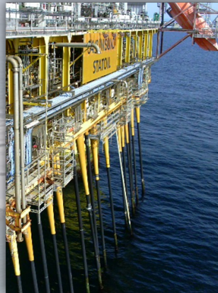
Dynamic Risers installation (close to 100 pull-ins)
