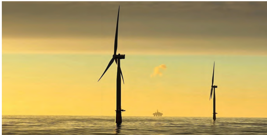
Late 2022 Equinor started producing power from the first installed floating turbines of Hywind Tampen's eventual eleven units. Photo courtesy of Equinor.
