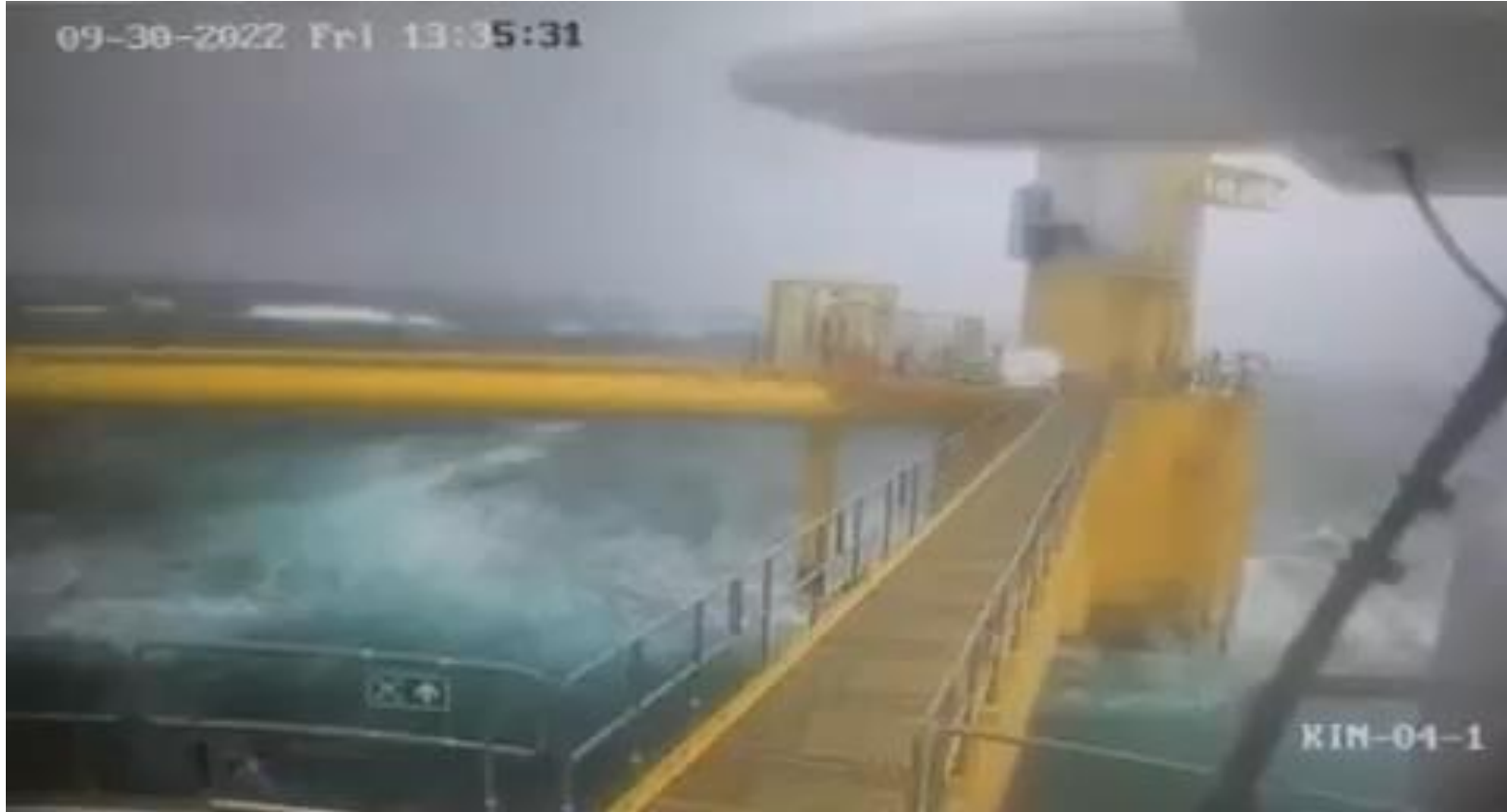
KIN04 Exposed to 8m Hs during a storm in Sept. 2022
