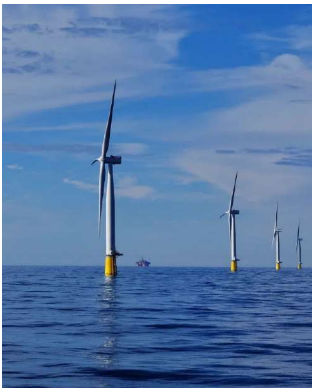
Hywind Tampen. Producing 94.6MW its 11 floating wind turbines (SPARs). The world's first full-scale electrification project. Photo courtesy of Equinor
